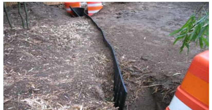
Figure 2: Barrier for Bamboo Containment
