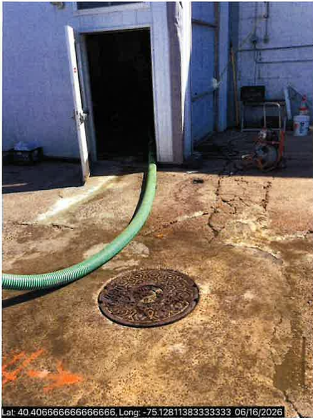
Photo #1 Hose leading inside to underground storage tank.
