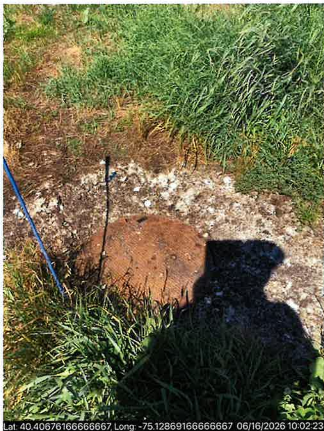
Photo #5 Manhole cover over underground storage tank opening.
