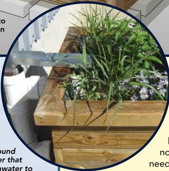
*Above-ground box planter that allows rainwater to flow through from the downspout*
